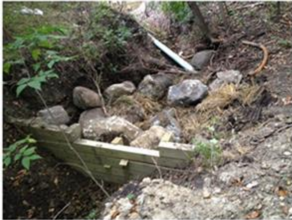
Picture #4: Log Crib Backstopped with Rock
