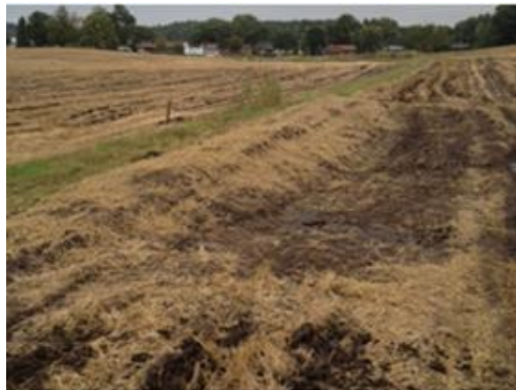
Picture #5: Erosion Control Berm in the Field
