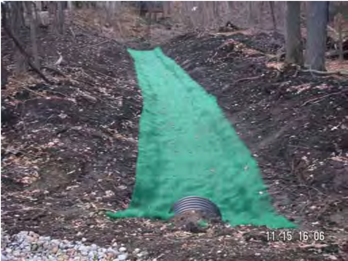
Figure 16. - Culvert Inlet, Looking West
