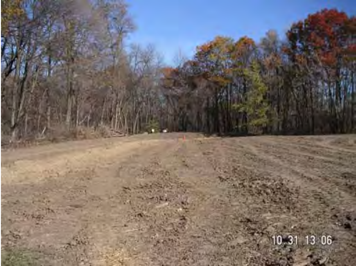
Figure 12. - Basin 4, Looking East, Wide View
