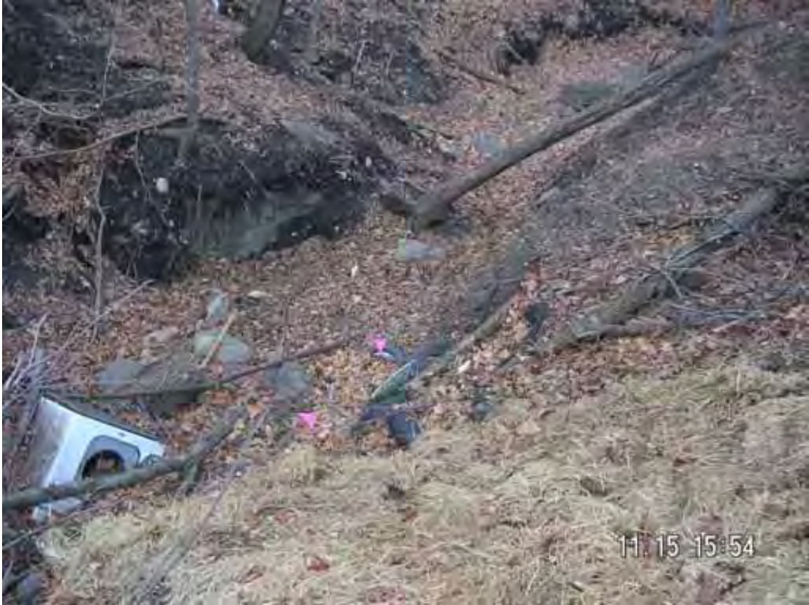
Figure 15. - Basin 4 Outlet, Looking Northeast
