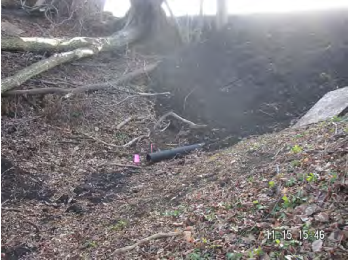
Figure 14. - Basins 2 & 3 Outlet, Looking Southwest
