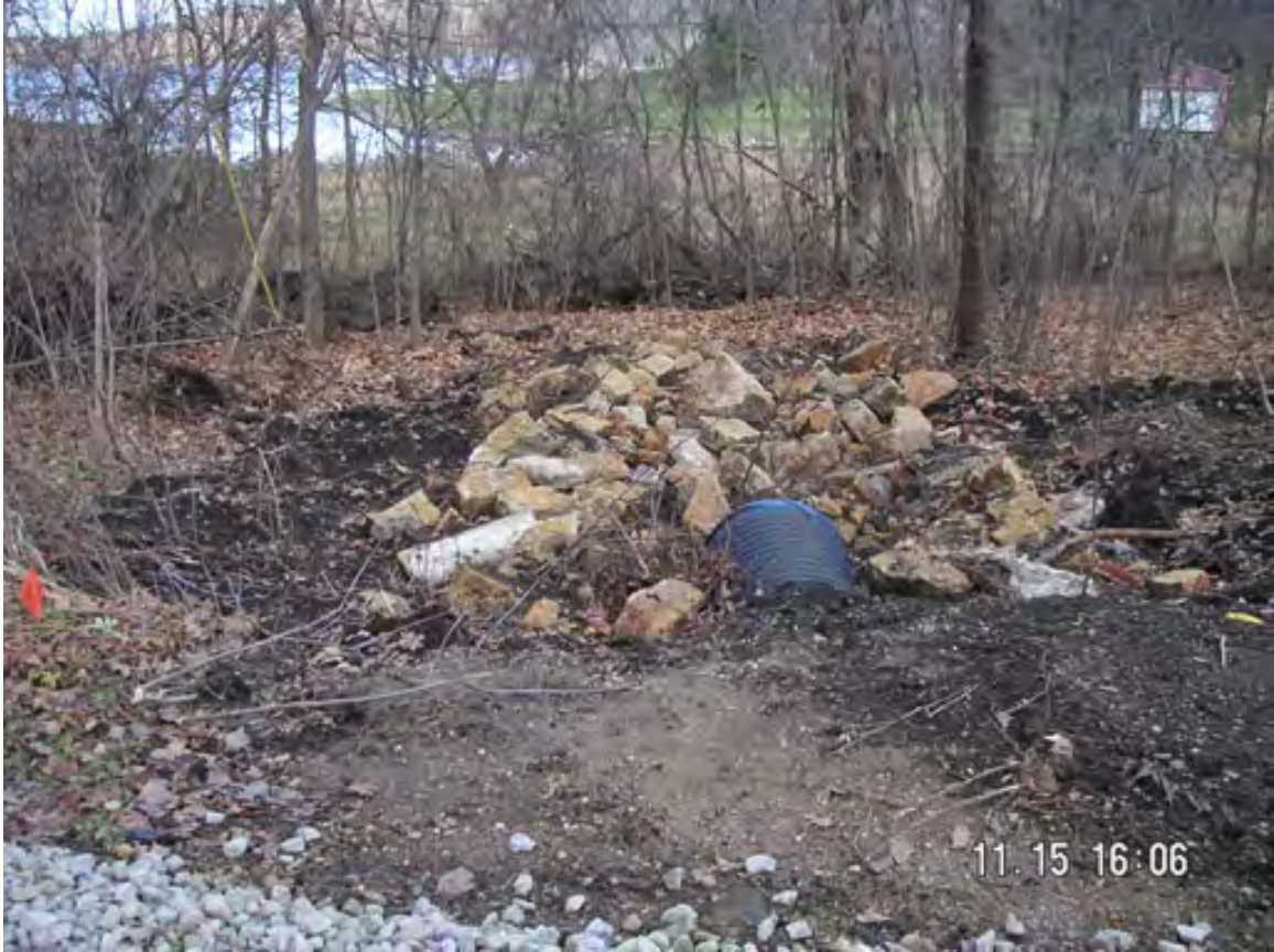
Figure 17. - Culvert Outlet, Looking East, Showing Wetland and Creek Mouth
