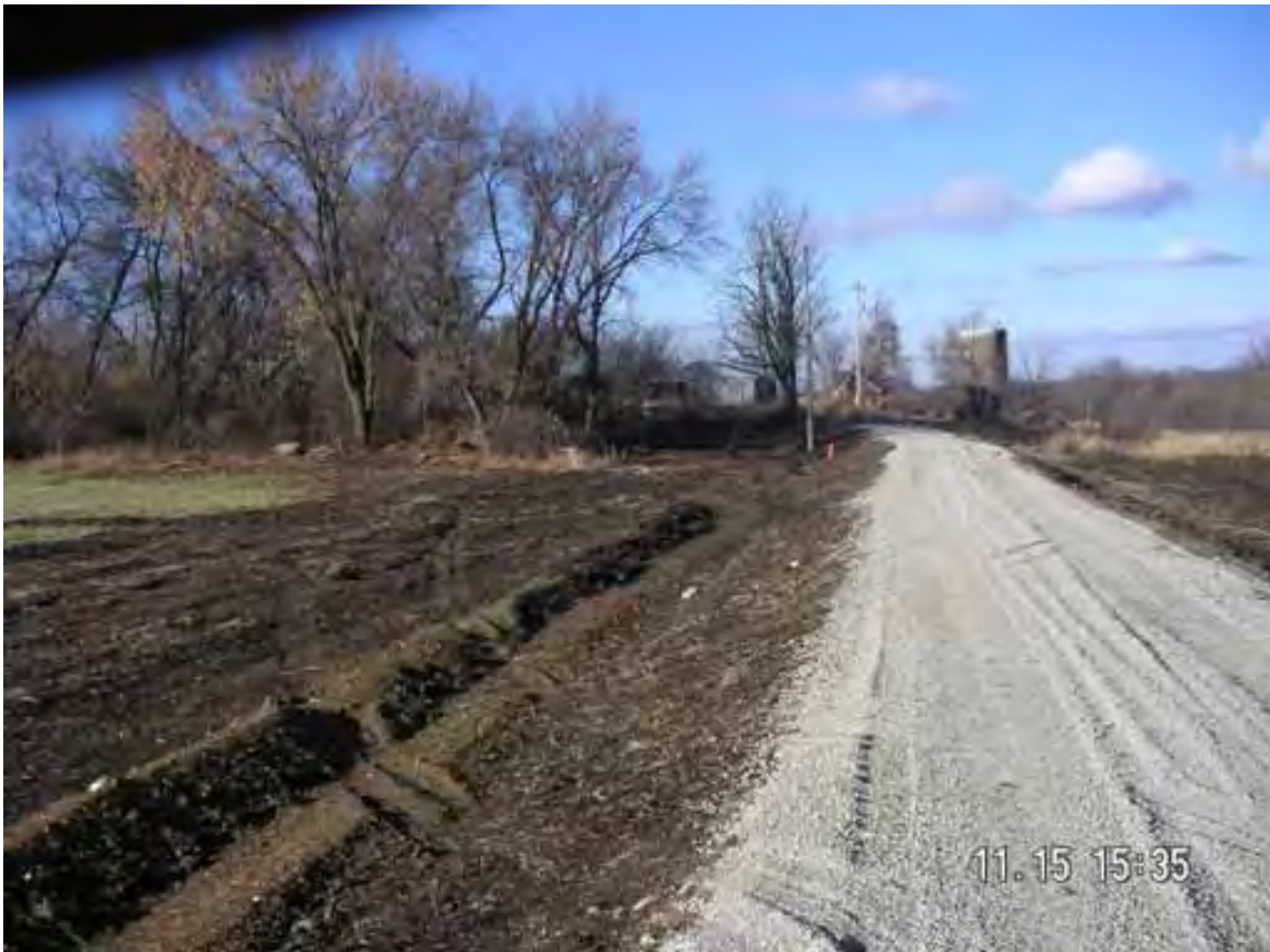
Figure 5. - Basin 1, Looking North
