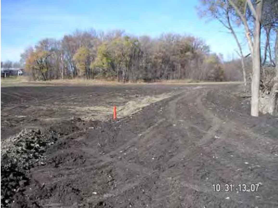
Figure 9. - Basin 3, Looking North
