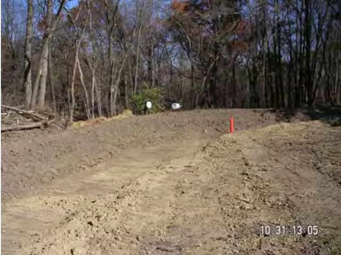
Figure 11. - Basin 4, Looking East
