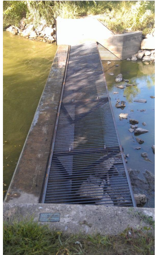
Figure 1 - Wolf Creek Fish Barrier
